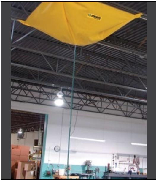
Suspended funneling design diverts damaging water from ceiling leaks to protect personnel, inventory, and equipment.
