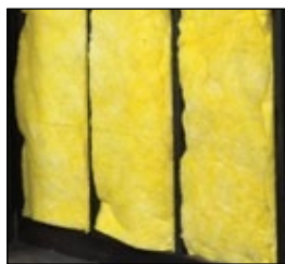
R-11 insulation in walls, ceiling, and sump walls
