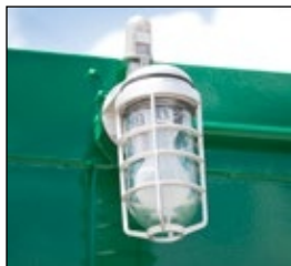
Vapor-resistant exterior light with photocell
